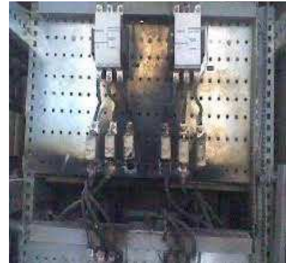
Burning of Fuse/MCCB/Cables due to harmonics (high heating)
